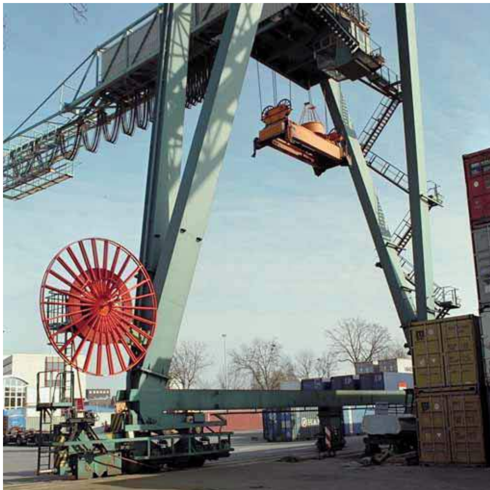
VAHLE Cable Festooning System for Container Crane Electrification.
